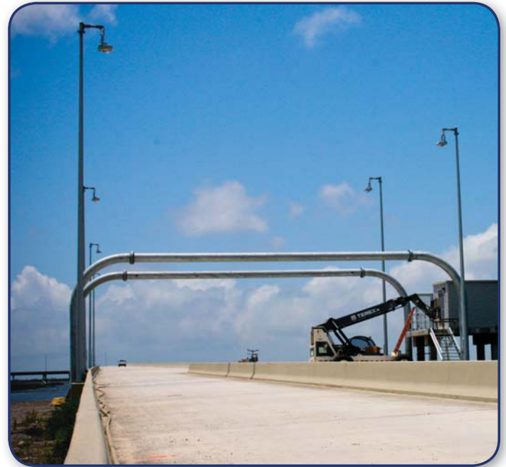
Bayou LaFourche electronic toll collection gantry.
